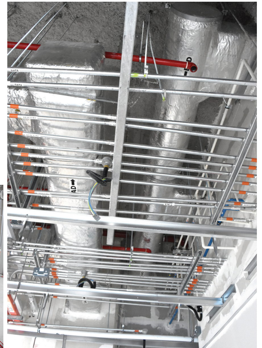
(Main) Schematics on how negative pressure is achieved in each room. (Above left and right) Engineers testing air tightness; airflow system during construction phase.
