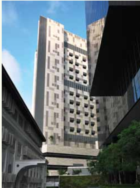
» The sharp and modern façade of the robustly designed National Centre for Infectious Disease (NCID) (middle) etches a sharp backdrop between the beautifully restored Palladian-style Heritage Building (left) and the Clinical Sciences Building of the NTU-Imperial College Lee Kong Chian School of Medicine (LKCMedicine) (right) in the Novena HealthCity Campus. The Heritage Building was formerly Nursing Quarters and later Administrative Offices for TTS before becoming the proud headquarters of the LKCMedicine.
